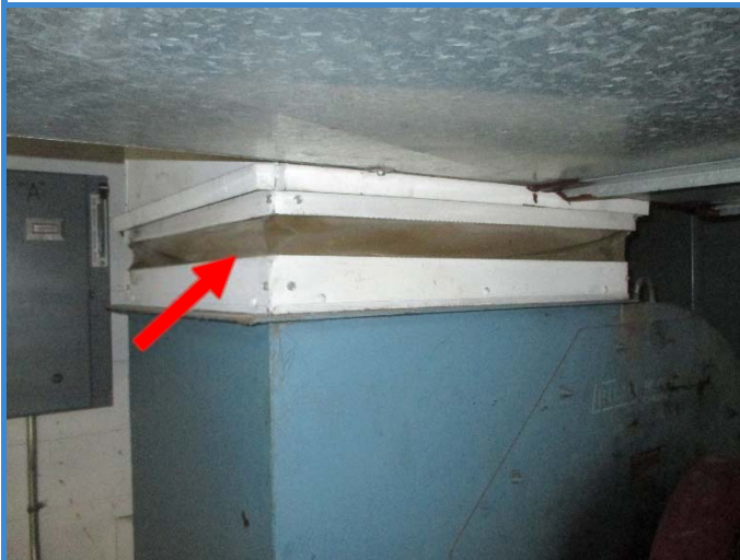
Photo 3: Typical view of the presumed ACM vibration dampers (see arrow) that were observed in the subject building.
