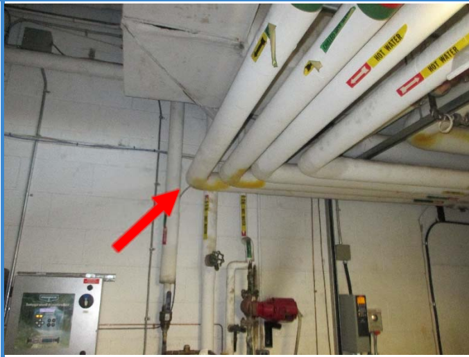
Photo 1: Typical view of the ACM parging cement fittings (see arrow) that were observed in the subject building.
