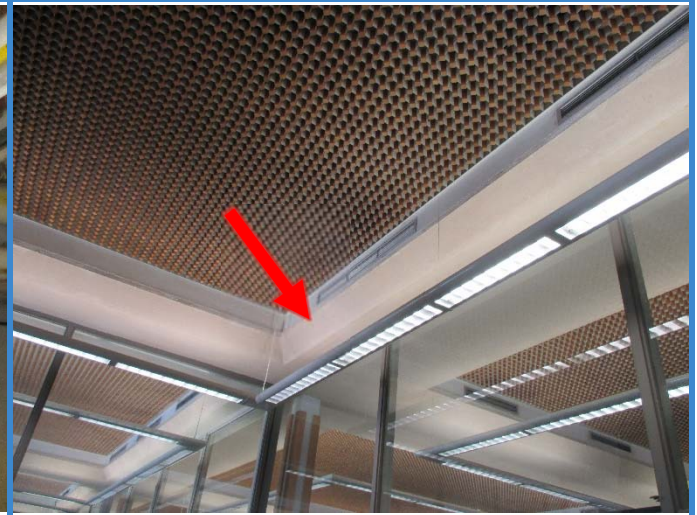
Photo 2: Typical view of the ACM texture coating (see arrow) that was observed in the subject building.
