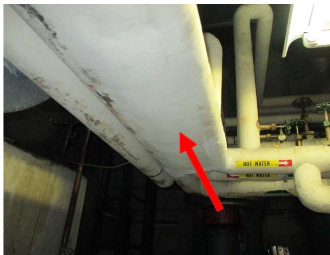
Photo 6: View of the ACM wrap packing (see arrow) that was observed in the subject building.
