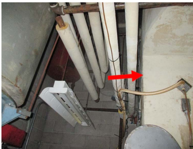
Photo 5: Typical view of the ACM duct paring cement (see arrow) that was observed in the subject building.
